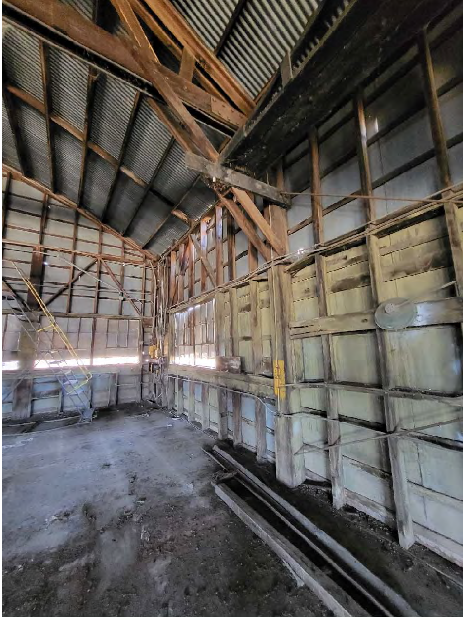
BUILDING 249 – BOWSTRING TRUSS TYPICAL CONNECTION
